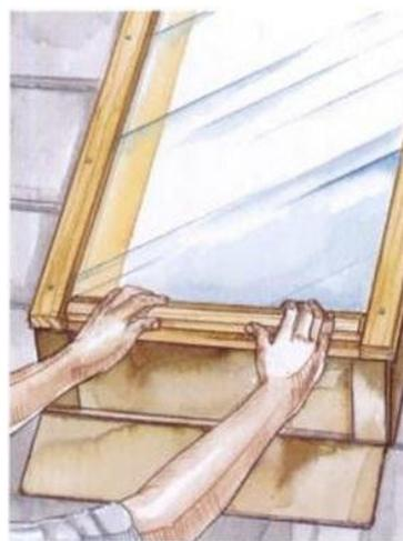
Lay the glass into the skylight frame and secure it with redwood stops. Use a beveled stop for the bottom piece.
