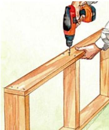
Assemble the window frames with screws. Add a 2 × 4 mullion in the center of the side window frame.
