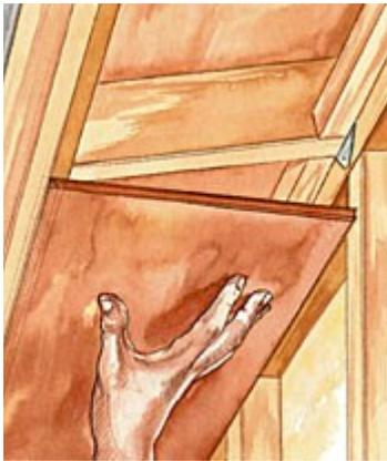
Rip the soffit panels to fit between the wall plates and fascia. Fasten the panels to the nailers, rafters, and subfascia.
