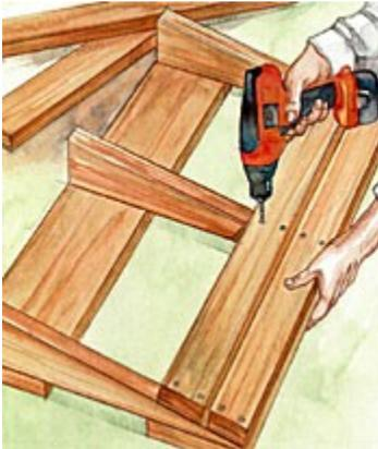
Build the ramp with pressure-treated 2 × 8s and 2 × 4s, following the plan's size or building it to a custom size.
