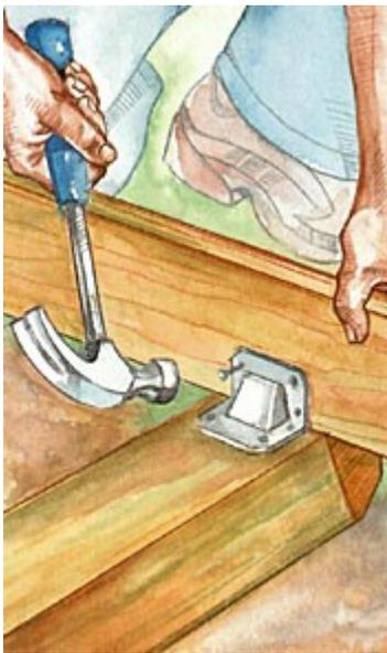
Secure the joists to the outer skids with angles. Drive hanger nails into the joists and 16d nails into the skids.
