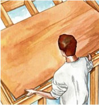
Install the plywood roof sheathing after installing the fascia. Nail every 6" at the edges and every 12" in the field.
